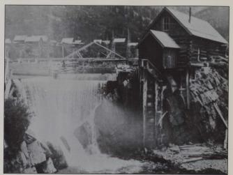
The Crystal Mill. One of the most photographed buildings in Colorado, the Crystal Mill was built about 1882 to provide power for the Sheep Montain Tunnel, one of the largest mines in Crystal City. The camp was founded in 1882 to thecause of its remote location south of Marke, never had more than several handred residents and was largely abundoned by 1910. Aspen Historical Souper Mistorical South
